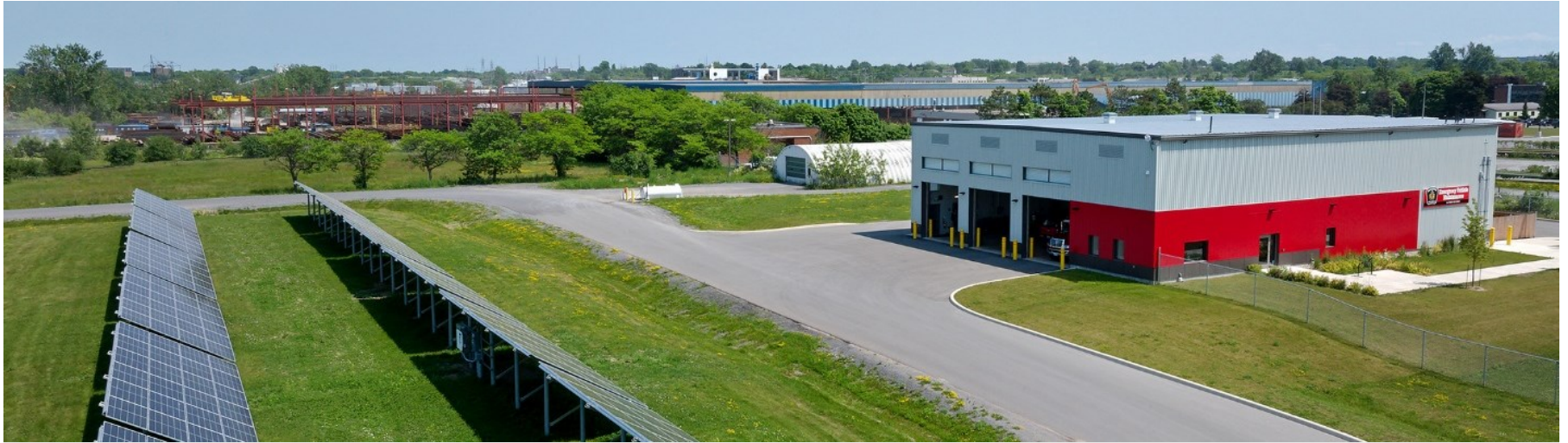
Figure 20. New Kingston Fire & Rescue Maintenance Garage
