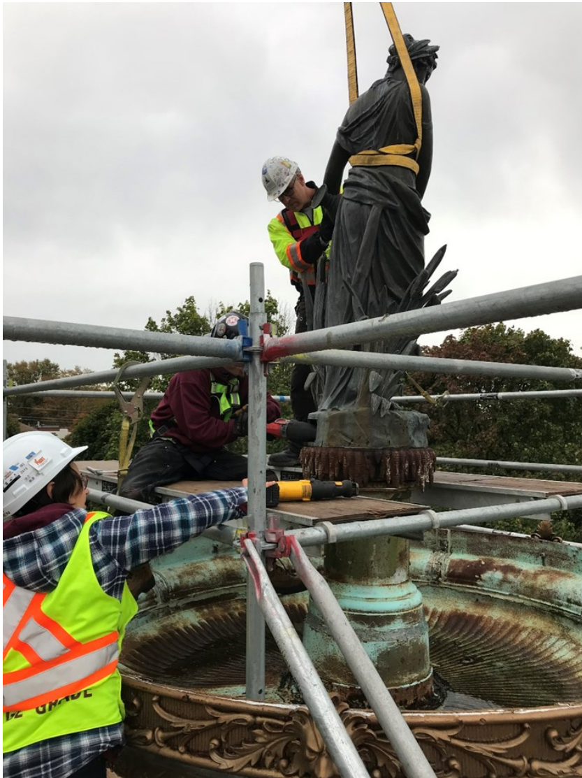
Figure 8. Disassembly of Kirkpatrick Fountain for Restoration (Frontenac County Courthouse)
