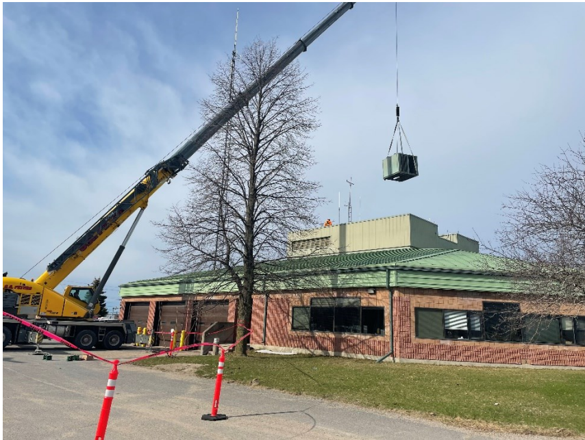
Figure 17. Kingston Fire & Rescue Headquarters During Installation of New Cooling Equipment
