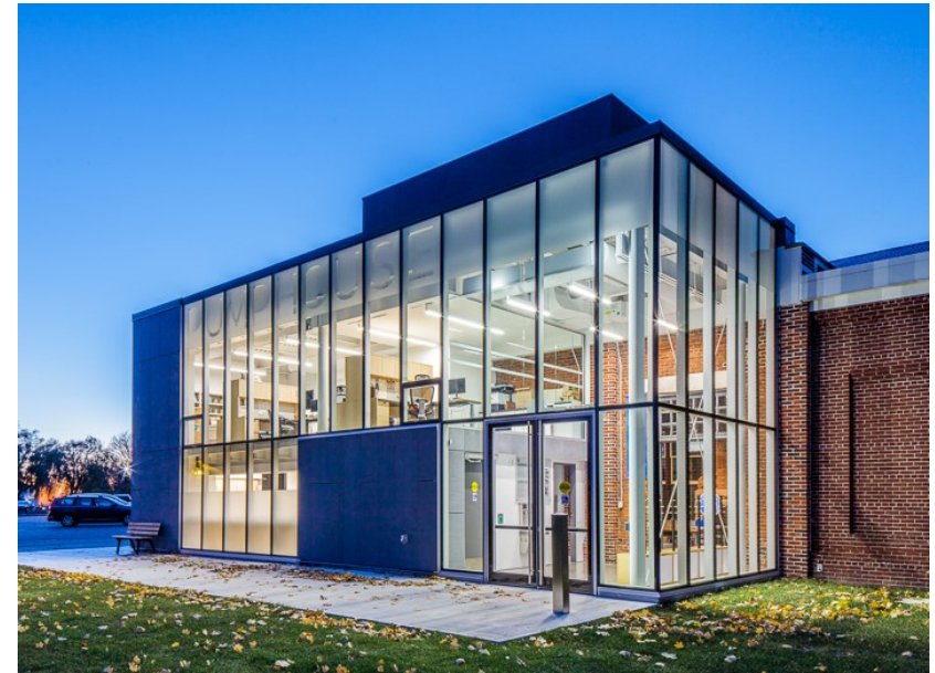
Figure 13. PumpHouse Museum Addition
