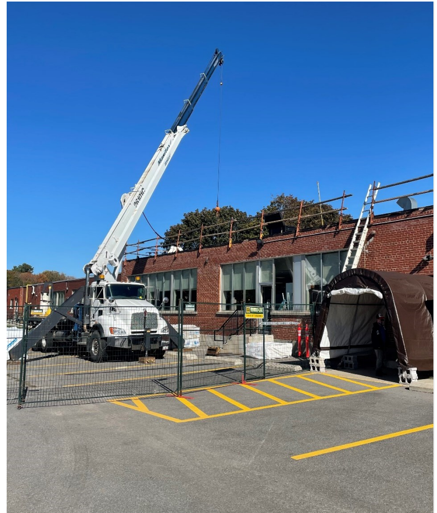
Figure 16. Kingston Senior's Association During Roof Replacement
