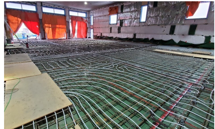
Figure 4. New Fleet Maintenance Garage Under Construction
