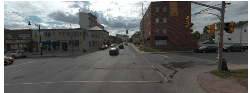
Figure 11. Example of Very Poor Road (OCI 20-0)
