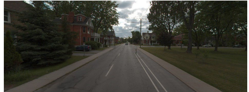
Figure 11. Example of Very Poor Road (OCI 20-0)
