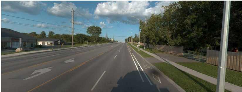
Figure 8. Example of Good Road (OCI 80-61)
