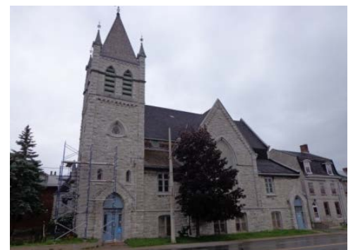
Ongoing alteration work-former Queen Street United Church
